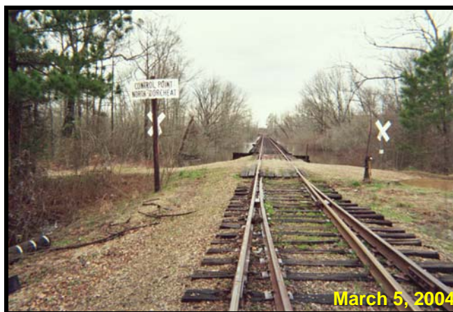
Photo 2: Looking west at the Alternative 4 crossing of Bayou Dorcheat
