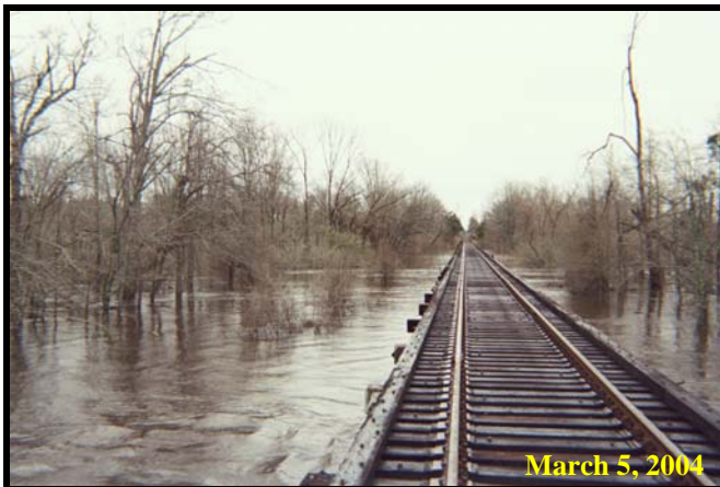
Photo 1: Looking east at the Alternative 4 crossing of Bayou Dorcheat
