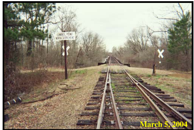
Photo 2: Looking west at the Alternative 4 crossing of Bayou Dorcheat
